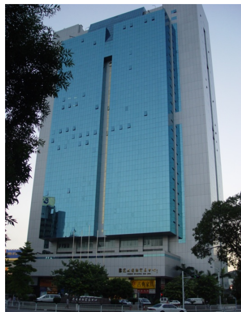
Fig. 1. Office building Housing Companies in Bangalore
